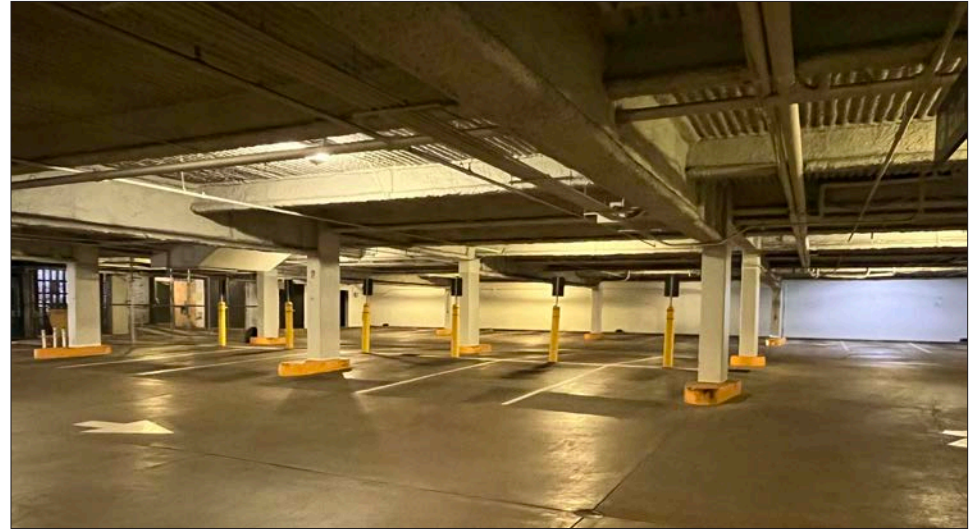
Secure 35 Car Parking Garage
